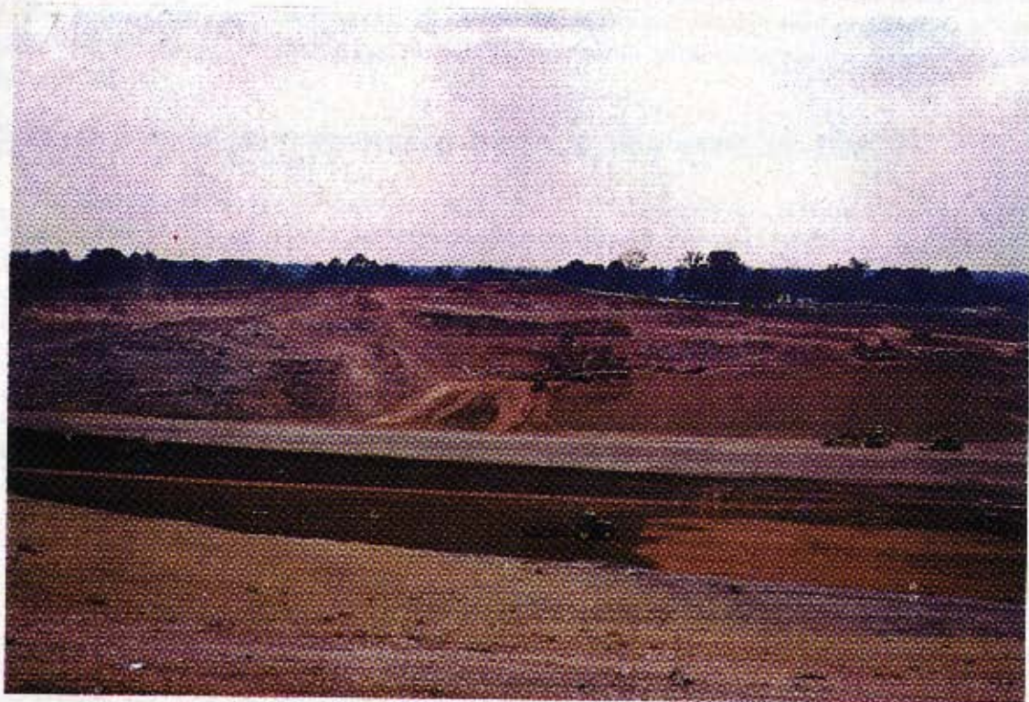
SANITARY LANDFILL SITE UNDER PREPARATION
